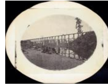
Photograph, Tennessee River Bridge 1st Michigan Engineers (126812.5)
