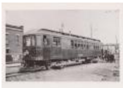
Photograph, Grand Rapids, Grand Haven and Muskegon Railway (2018.5.30)
