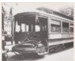
Photograph, Damaged Streetcar (2018.5.40)
